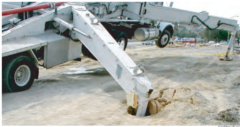
Figure 14 Hidden voids cause accidents
